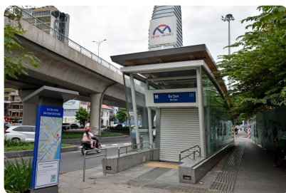
Metro station in Ho Chi Minh City.
